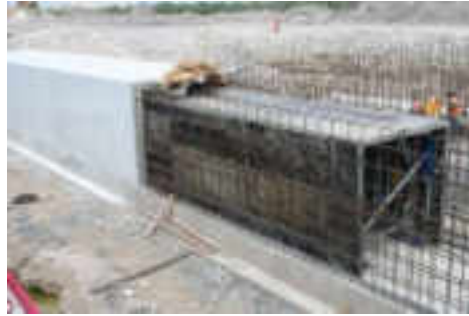
Figure 3-1: Reinforced Concrete Box Culvert
