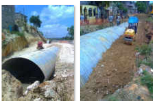
Photo 3-1: Metal Pipes installed in Phase I of the Project, like those to be used in Phase II.
