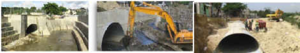
Photo 1-3: Canal Buenos Aires Works
