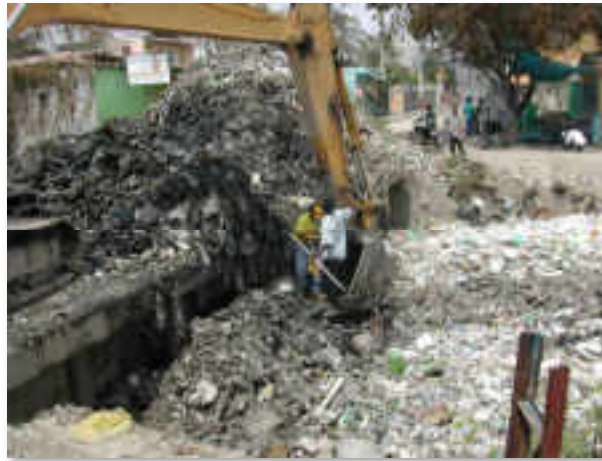
Photo 4-4: Canal Cleaning in Phase I of the Project
