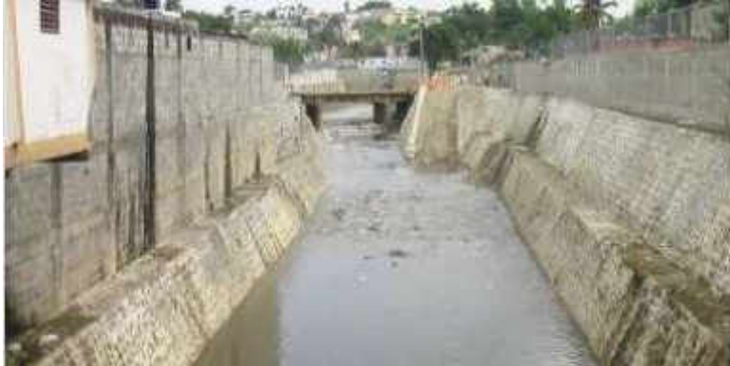
Photo 4-6: Re-profiling of the Guajimía Canal in the Section from 400 m Upstream of the Guajimía-Buenos Aires confluence to the 6 de Noviembre Highway Bridge that was executed as part of Phase I of the Project
