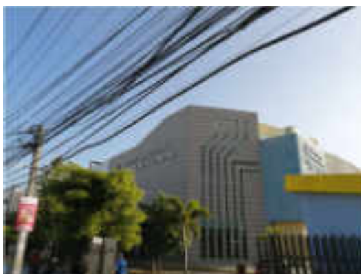
Photo 6-9: Marcelino Vélez Hospital, in the municipality of Santo Domingo West
