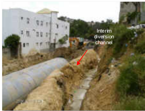
Photo 4-5: Diversion Channel used during Phase I of the Project
